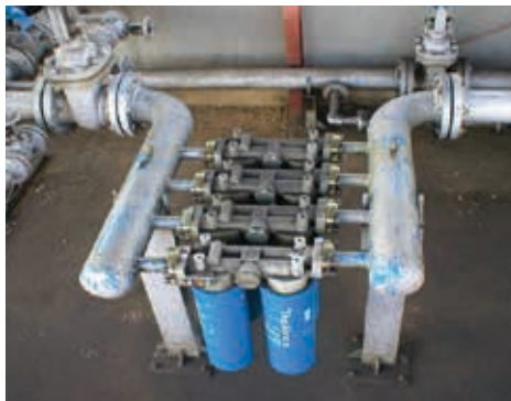
Single-pass Bulk Fuel Filtration System
